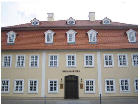
The “Old Pädagogium” in Niesky, now a public library, built in 1741 as the first parish house of the newly founded community in Niesky. Between 1760 and 1945 it was used as an advanced boarding school.
